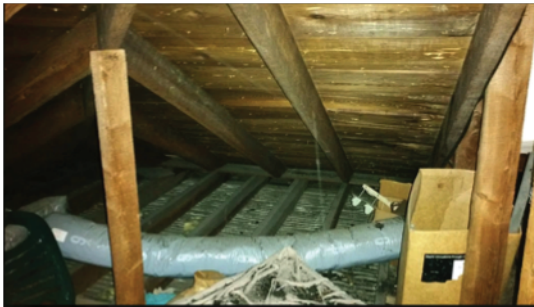
Before attic insulation
