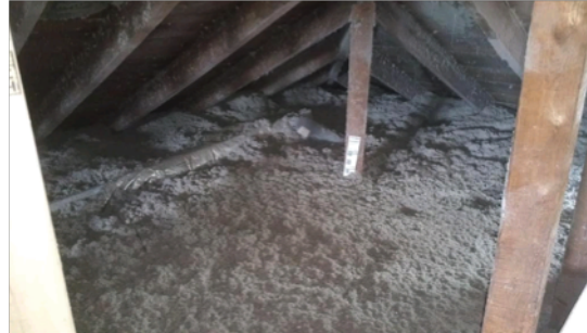
After attic insulation
