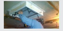
Radiant tube heaters are a more efficient way of warming the birds. Instead of heating the air, radiant heaters direct heat to the objects in the house such as the walls, floor and chickens.
