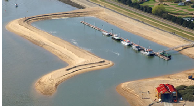
Figure 6 The standalone jetty for the Sheringham Shoal wind farm.
