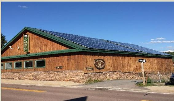
This 30,866 kWh solar array mounted on a creamery and market roof at FireFly Farms powers a goat cheese production farm.
