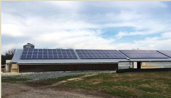
Solar PV systems must be sized appropriately for the site conditions and the needs of the farm. On Sarfraz Family Farm, a 69,300 kWh PV array powers a poultry operation.
