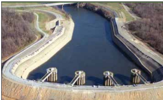
The Muddy Run Pumped Hydro Facility, originally constructed in 1966 and located along the Susquehanna River just north of Maryland, provides 1,070 MW of power into PJM.
